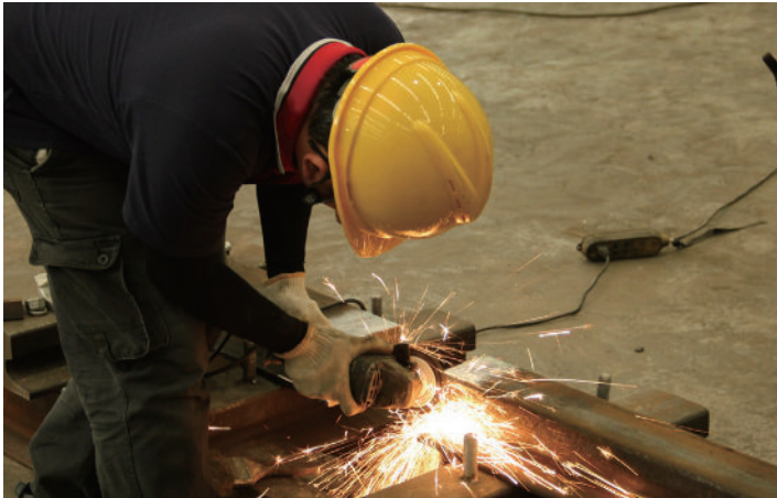
Inspect & clean up the rail end
