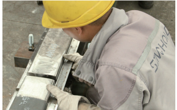
Alignment of rail ends
