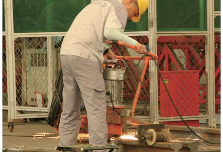
Demount the mold & remove the dross
